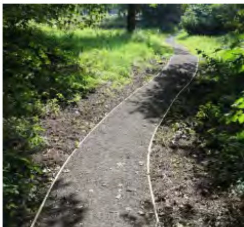
Upgraded new footpath
